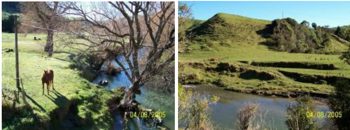
Figure 8. Makuri Stream showing lack of riparian fencing, full stock access, and bank erosion (2005).
