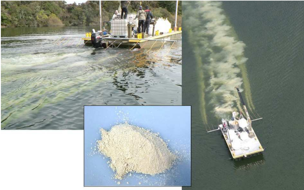
Figure 50. Application of fine granular Aqual P™ on Lake Okaro in August 2009. The product was injected as a slurry 3-5 m below the lake surface from a barge. Fine grain product in the inset.
