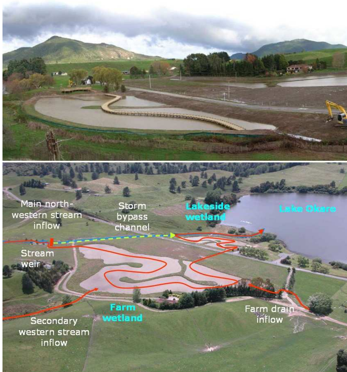
Figure 40. The constructed wetland at Lake Okaro at the time of construction. Top: Public access to the wetland is provide by a viewing walkway through the part of the wetland in the lake domain. Bottom: The stream water is forced to follow a convoluted flow path by the use of ridges within the
