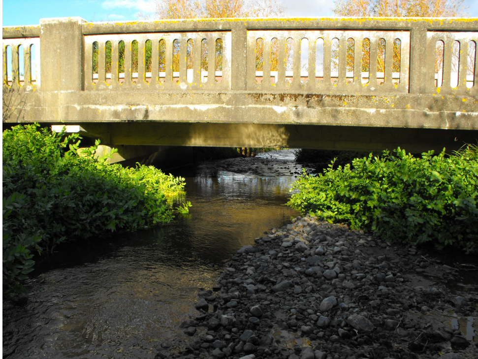
Photo 1. Bed aggradation at Kumeti Bridge over State Highway 2
