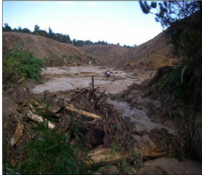
Figure 5: Erosion and debris problems as a result of undertaking large scale earthworks in association with forest to farm conversion operations in early winter
