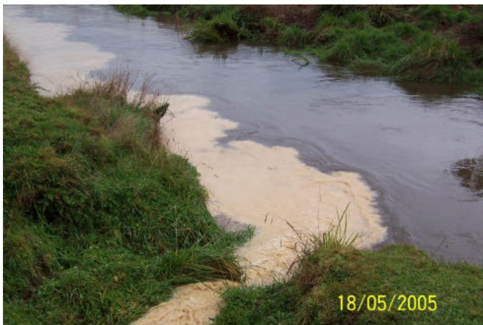
Figure 2: Discharge of sediment-contaminated stormwater from poorly managed earthworks operations in the Bay of Plenty
