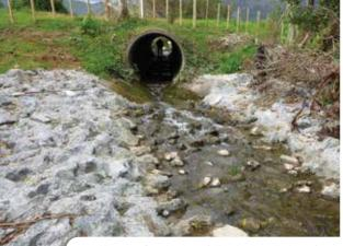
Kingston Road culvert following installation of rock ramp to enable fish passage
