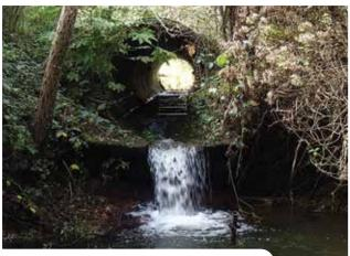
Kingston Road culvert with greater than 1 metre perch and undercut. Not fish passable
