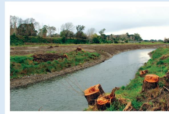
Stream clearing work along the Tutaenui Stream undertaken winter of 2021. Fencing and riparian planting will follow with a pathway meandering along the stream down to the Rangitikei River. Prior to this clearing the stream was clogged and overgrown – the large tree on the right was pulled out and was just one of many things impeding the stream's flow.
