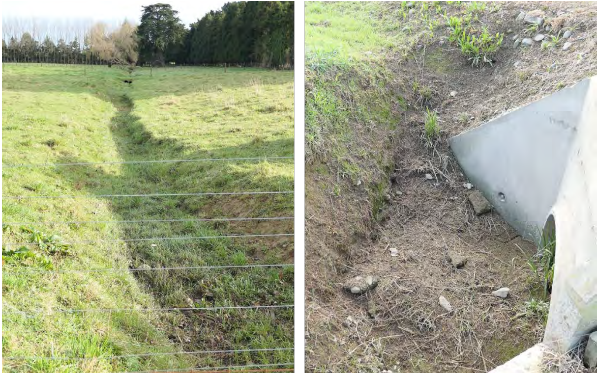
Figure 12. Undersized culverts and narrowing channel downstream of upgraded culvert (left). Upgraded culvert invert approximately 1.2 m below and perpendicular to downstream channel invert (right)
