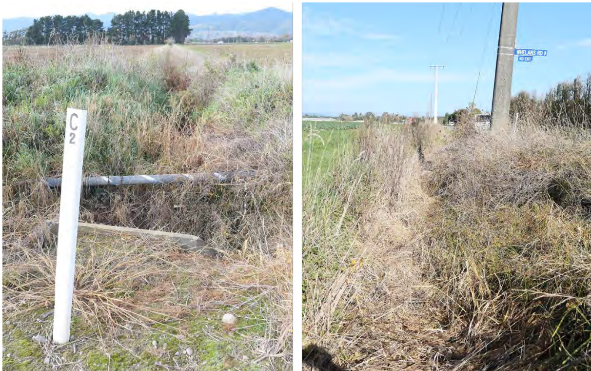
Figure 11. Examples of drainage network constraints due to vegetation growth in channels
