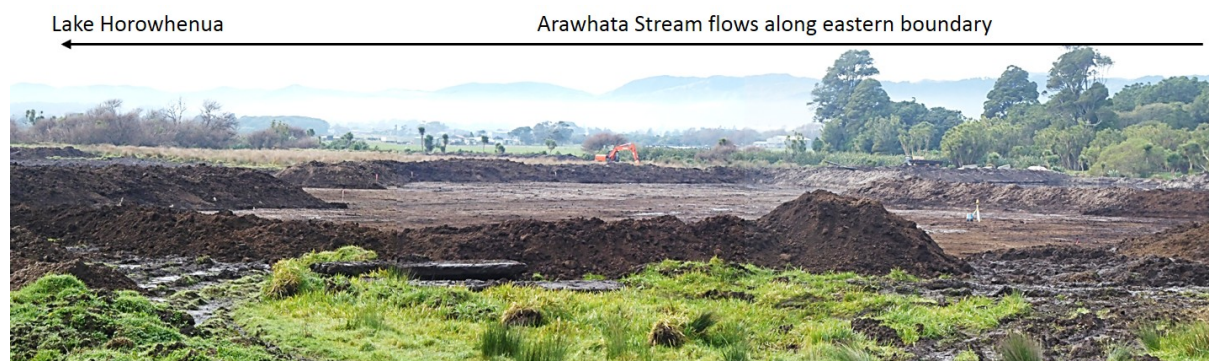
Figure 13: Construction of a large shallow sediment trap beside the Arawhata Stream. The Arawhata Stream flows along the eastern side of the trap and will flow into it when the water levels are high, allowing the sediment to settle in the slower moving water inside the ponding area. [Photo montage by Max Gibbs 22/06/2017].
