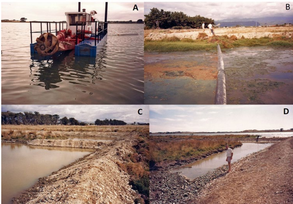
Figure 25: Trial dredging on Lake Horowhenua on 10th February 1989. Showing A) the dredge used, B) the pipeline delivery to shore, C) the on-shore dewatering pond and bund, and D) the dewatered sludge. [Photos by Max Gibbs].
