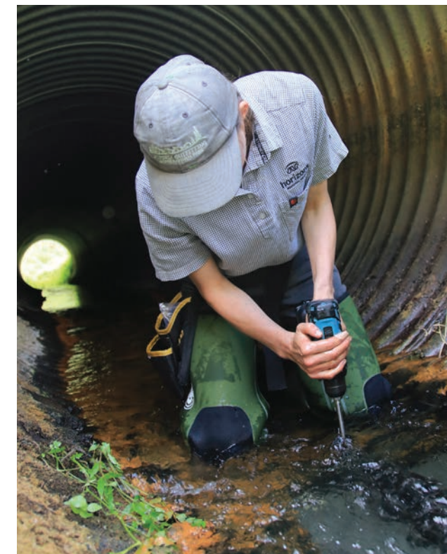
Horizons' Freshwater staff remediating a fish passage barrier by installing a mussel (spat) rope in a culvert.
