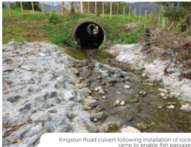
Kingston Road culvert following installation of rock ramp to enable fish passage
