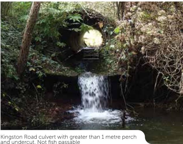
Kingston Road culvert with greater than 1 metre perch and undercut. Not fish passable
