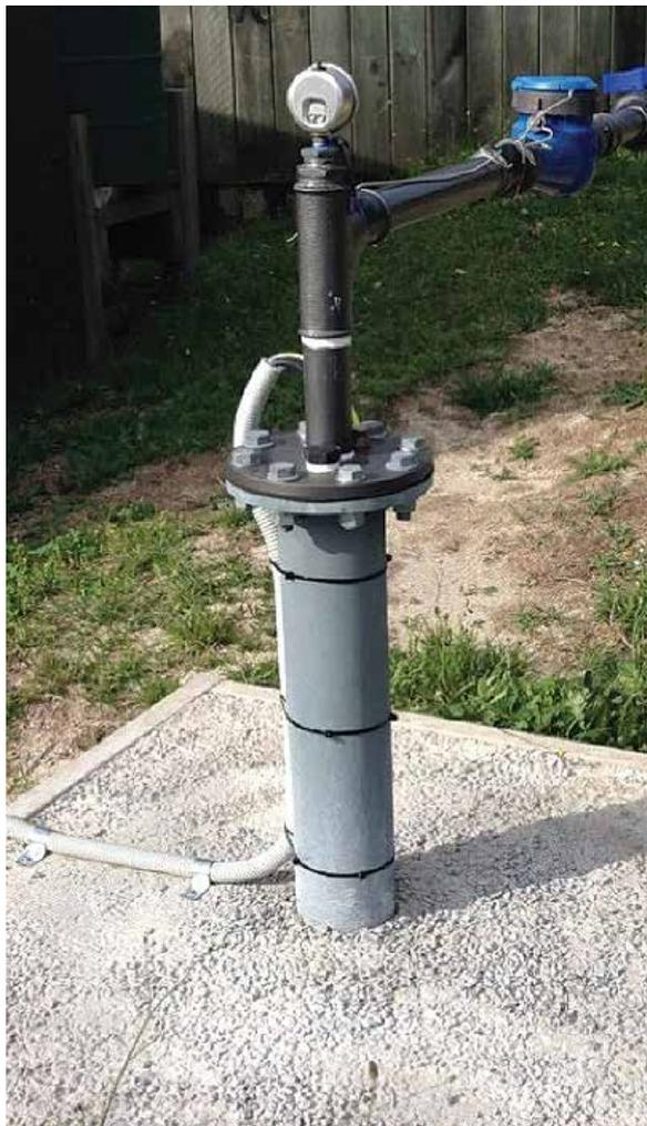
A secure groundwater supply requires a sealed wellhead, concrete pad and backflow prevention device, to reduce the risk of contaminants entering the bore
