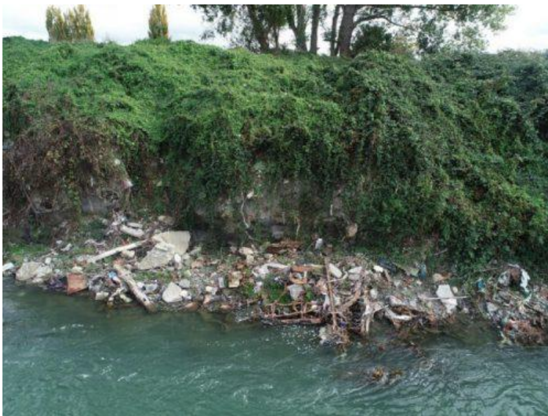
Figure 8.19: Exposed debris of Putorino Road landfill on the river bank of the Rangitikei river (2018) (Rangitikei District Council, 2020).
