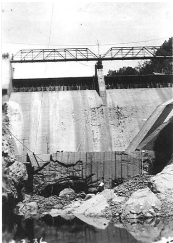
Figure 8.15: Damage to No.1 Dam in the 1936 floods (Kete Horowhenua, 2021).
