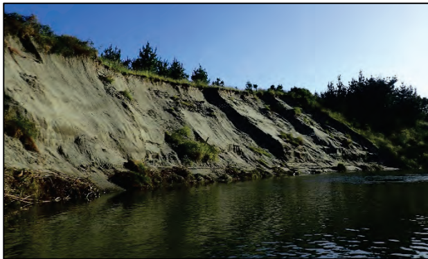
Ōhau estuary site T8, eroding sand dune mid-estuary
