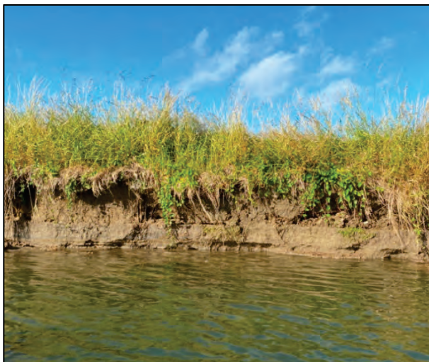
Eroding banks at site T7
