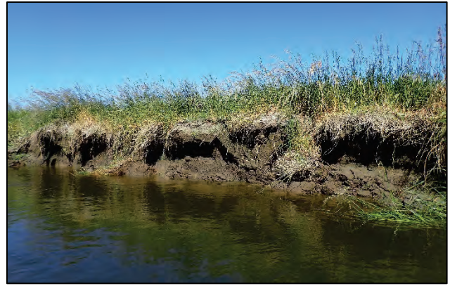
Bank erosion in the upper estuary
