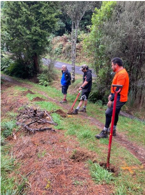
Photos above: Leo, Ti, Johnny and Dave of Ruapehu Worx not letting the wet weather halt work (though covid has) as they install the short boundary fence to protect the wetland from ingress by cattle, bikers or potential rubbish dumpers (probably how some of the weeds got there).
