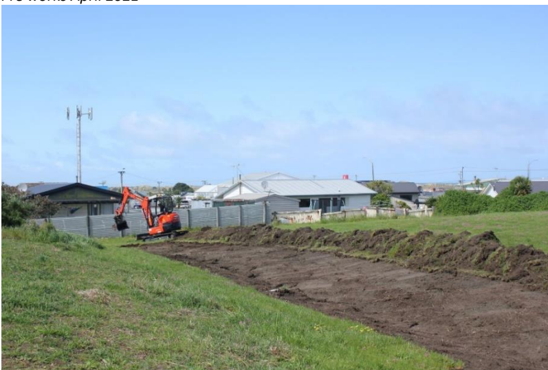
Preparing ground removing Kikuyu October 2021
