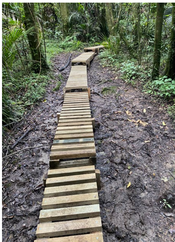
Figure 16: Track rafts at the Fern Walk.
