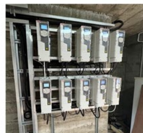
Newly installed variable speed drives for gate motor control
