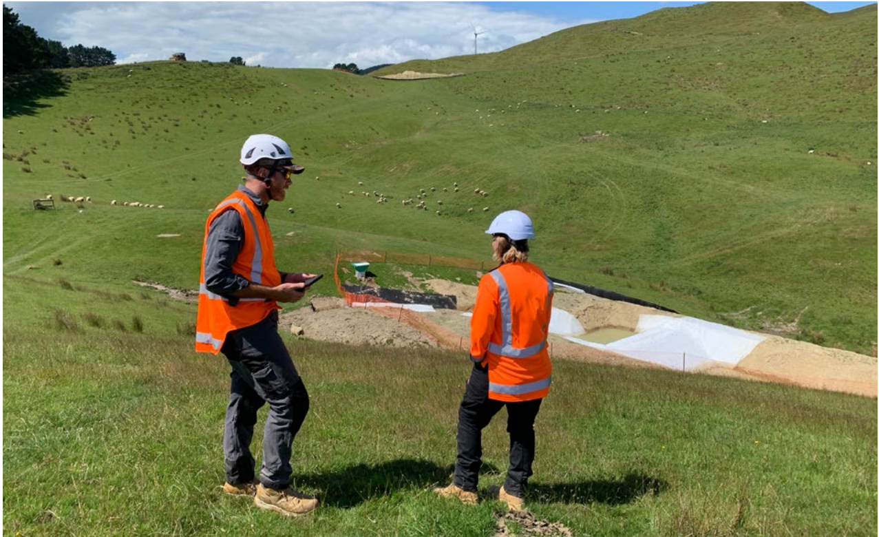
Regulatory staff inspecting a site
