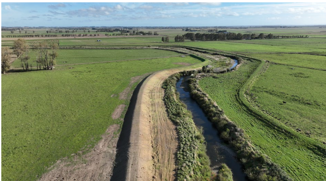
Newly built stopbank to provide flood protection
