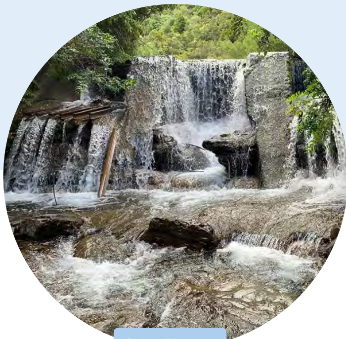
Barrier to fish passage
