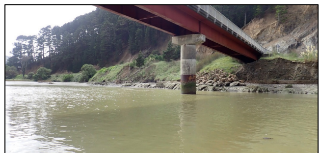
High turbidity waters at Akitio Bridge.
