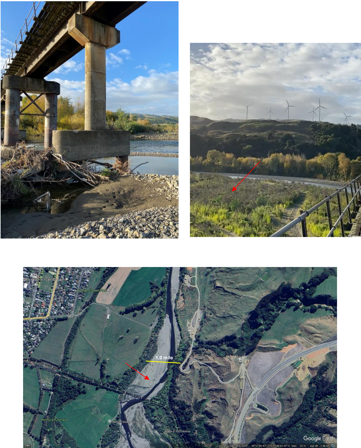
Figure D1: Railway Bridge
