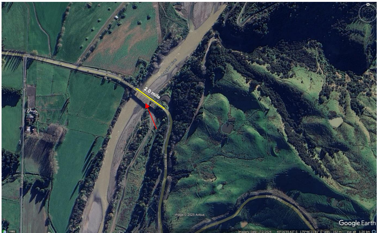
Figure D2: Saddle Road Bridge
