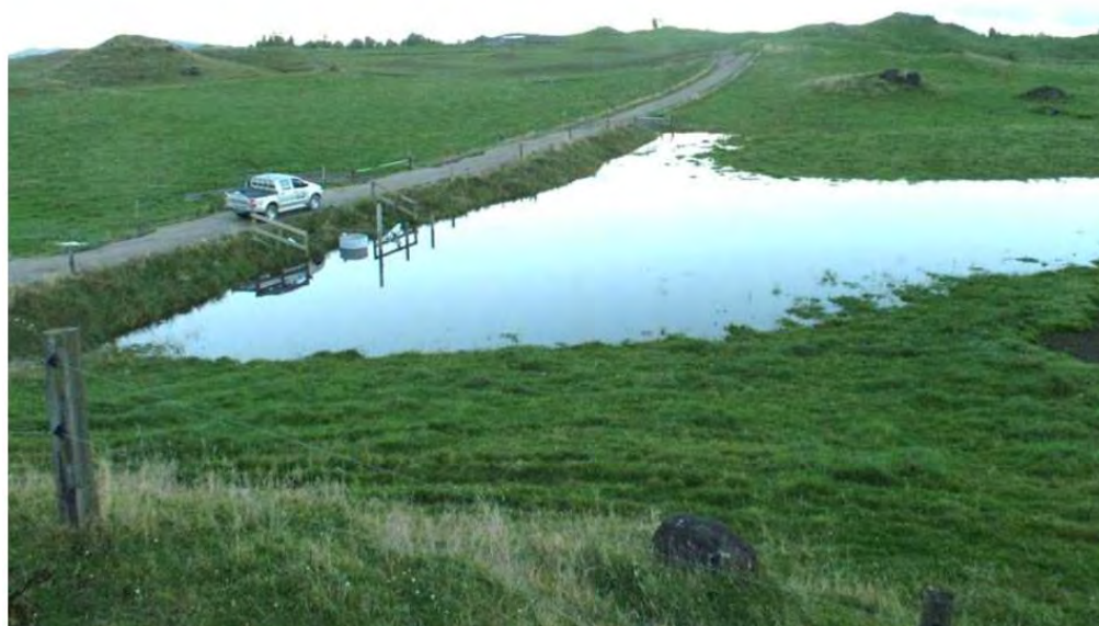
Figure 5: (Photo: Dylan Clarke) A typical detainment bund, designed to temporarily pond ephemeral stream water, Waiteti Stream catchment, Rotorua, March, 2012. This photograph has been taken after a runoff event and the pond is still draining.
