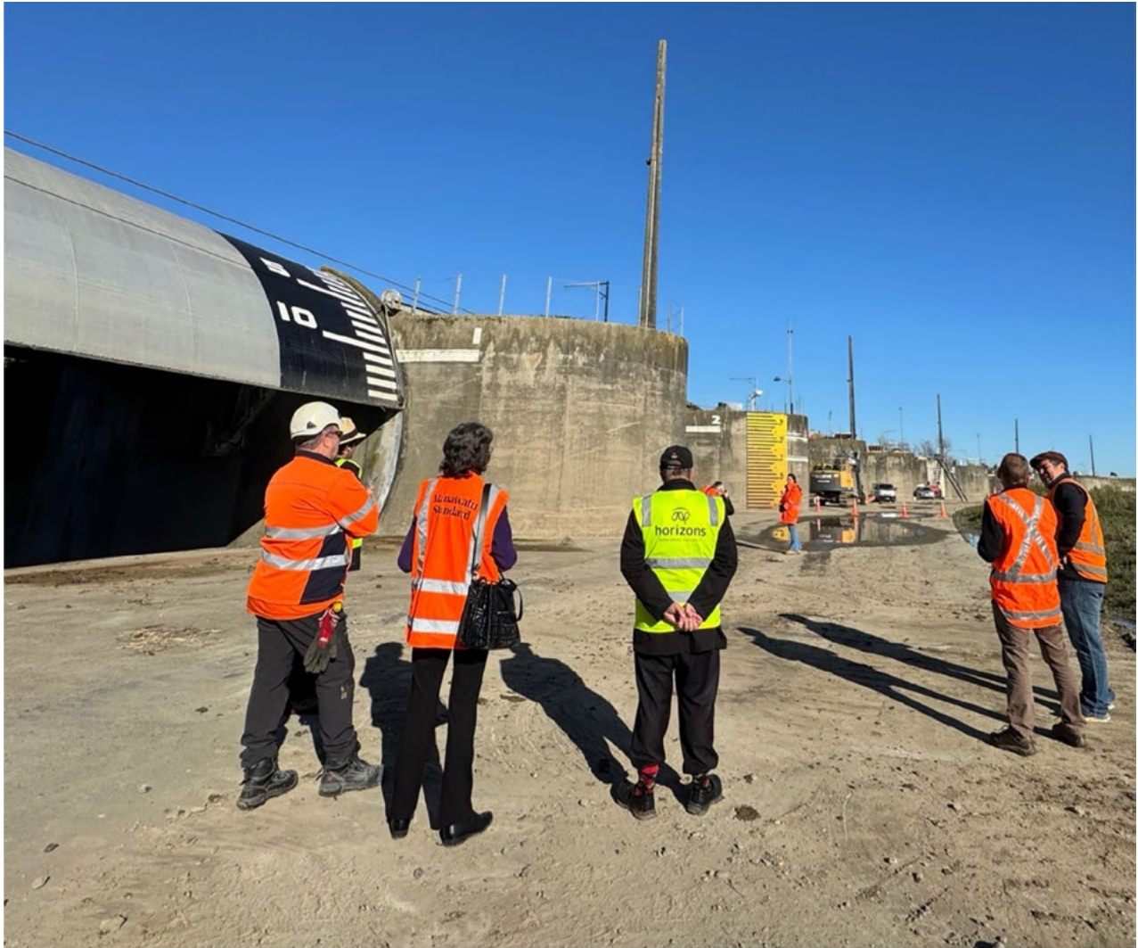
Media site visit at Moutoa Floodgates to view upgrade work in progress
