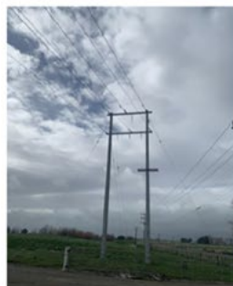
One of two new H-Structure poles for Overhead Lines
