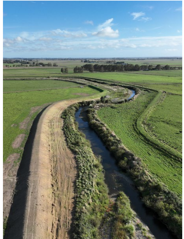
Newly built stopbank for flood protection
