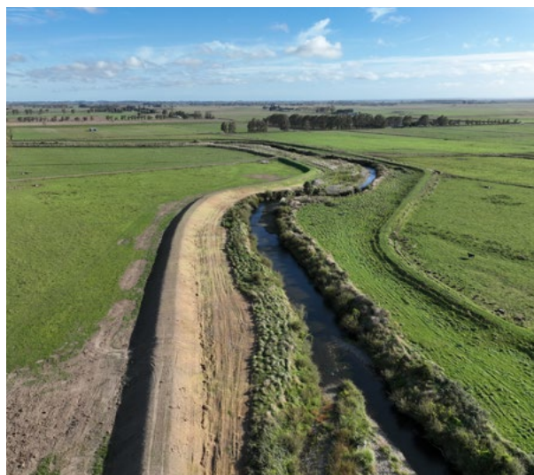
Newly built stopbank to provide flood protection
