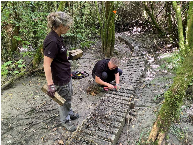
Figure 15: Staff carrying out track repairs
