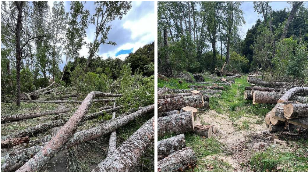
Figure 14: Pettifar Loop before and after track clearance works, February 2026
