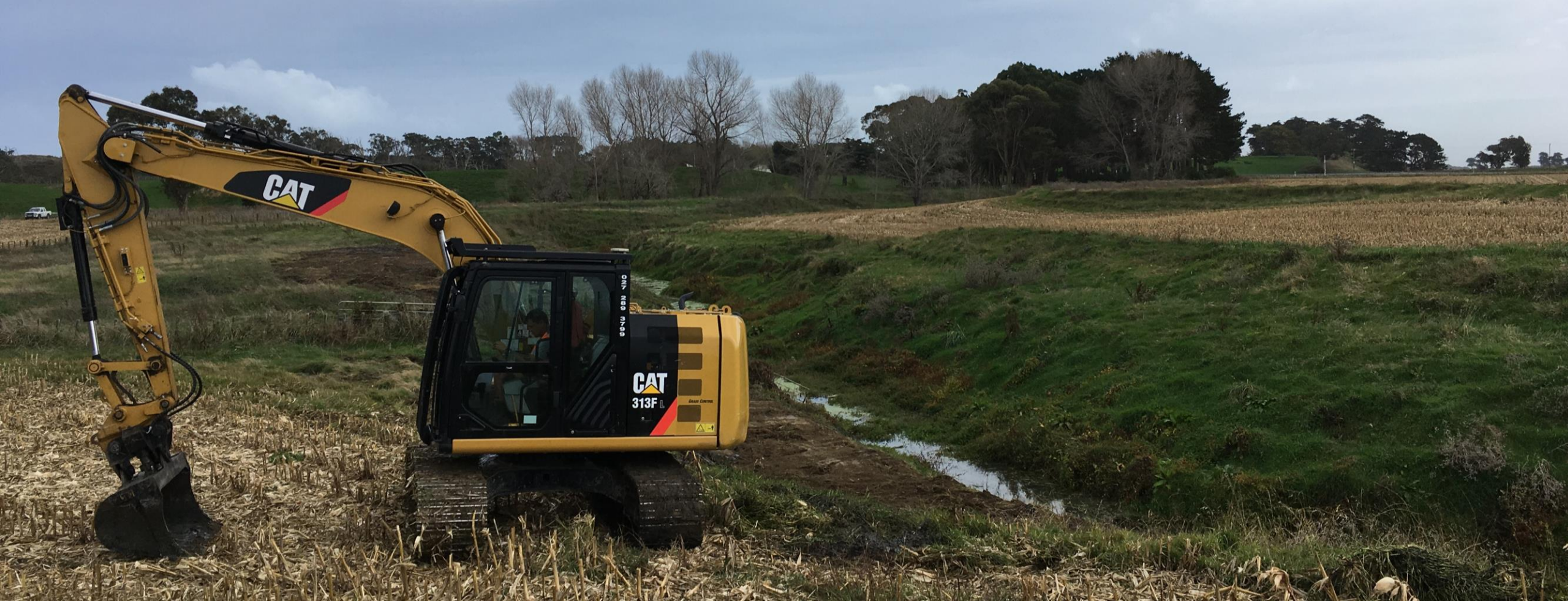
Photo – Makirikiri lower channel clearing
