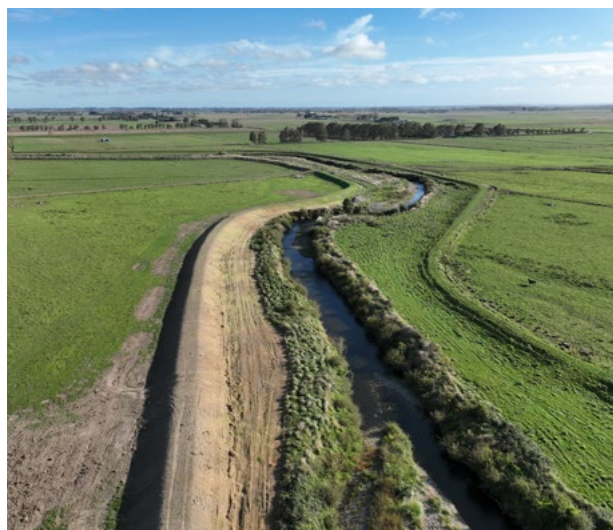
Newly built stopbank to provide flood protection
