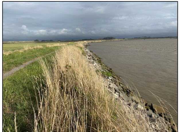
Armoured stop-banks prevent the landward migration of intertidal habitats in response to sea level rise.
