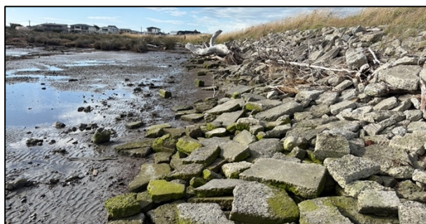
Rip-rap armouring of flood stop-banks is extensive along the true right of the lower estuary.
