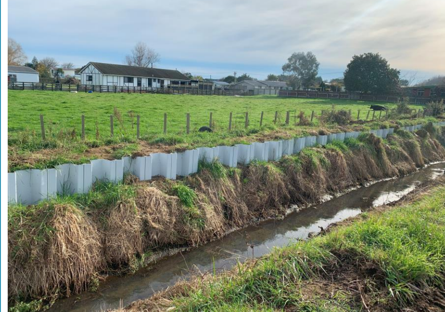
Sheetpile wall – Kings Canal, Foxton
