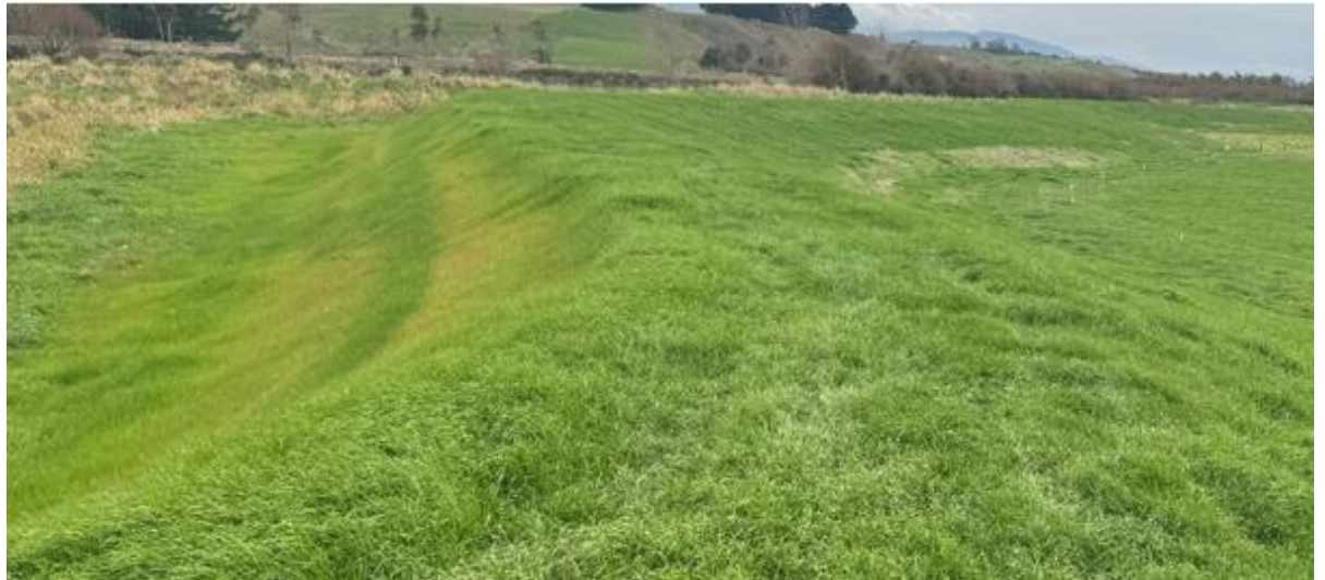
Photos: Upgraded stopbank in the Koputoroa
