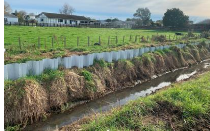
Sheetpile wall – Kings Canal
