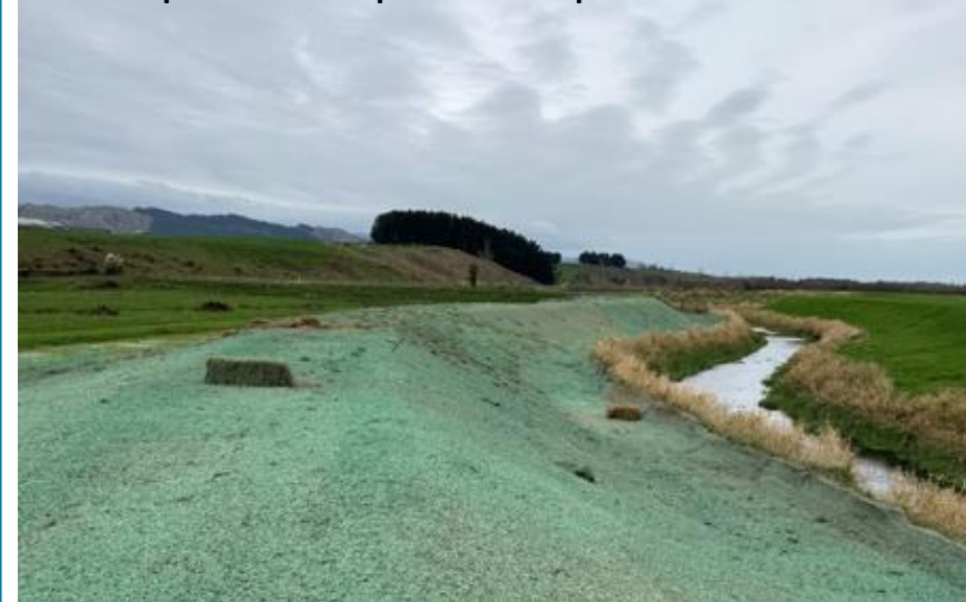
Completed stopbank Koputoroa Stream
