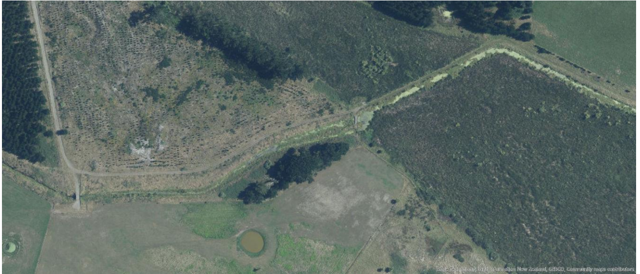
Figure 19: Drains and weir at north-west boundary of Pukepuke lagoon
