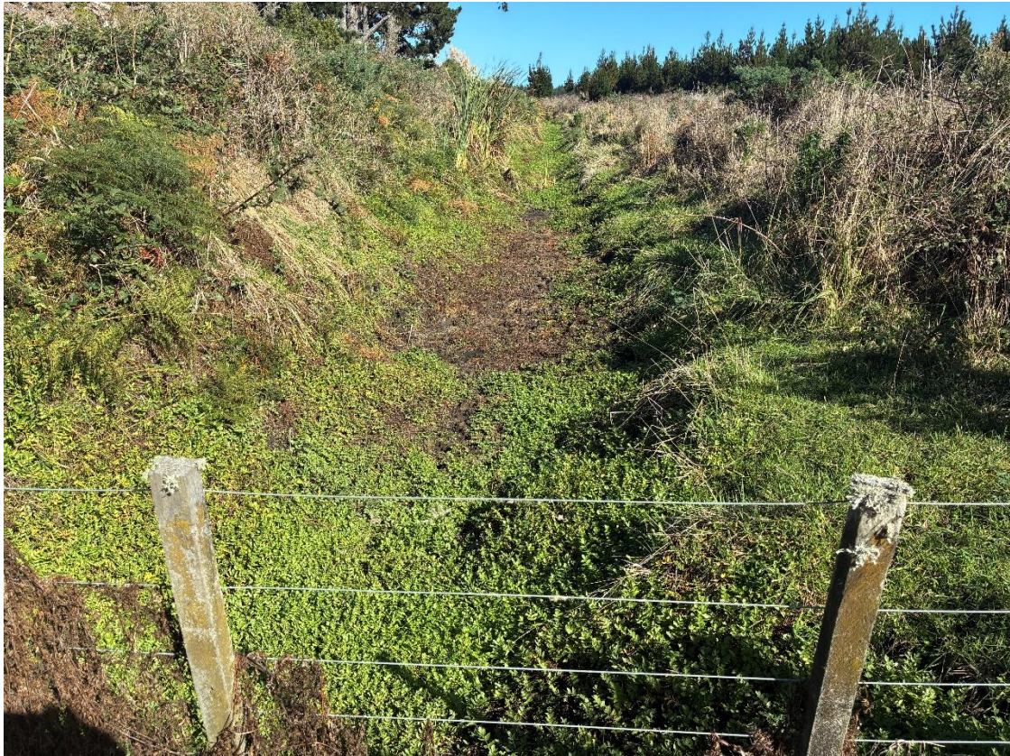
Figure 23: View along drain channel leading north-west away from weir
