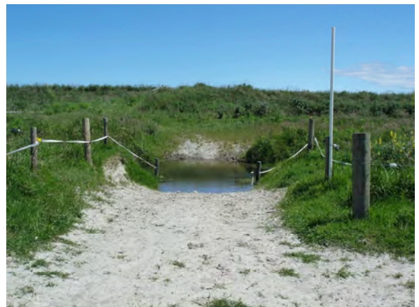
Stream crossing from the flood zone side of the stop-bank
