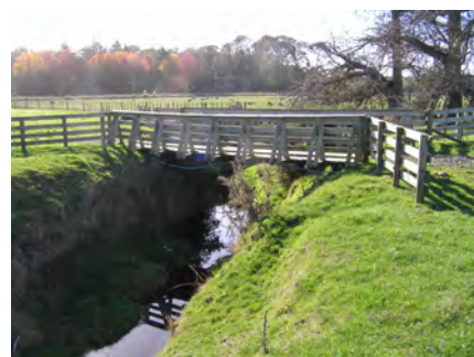
Bridge adjacent to the ford that crosses the non-perennial stream
