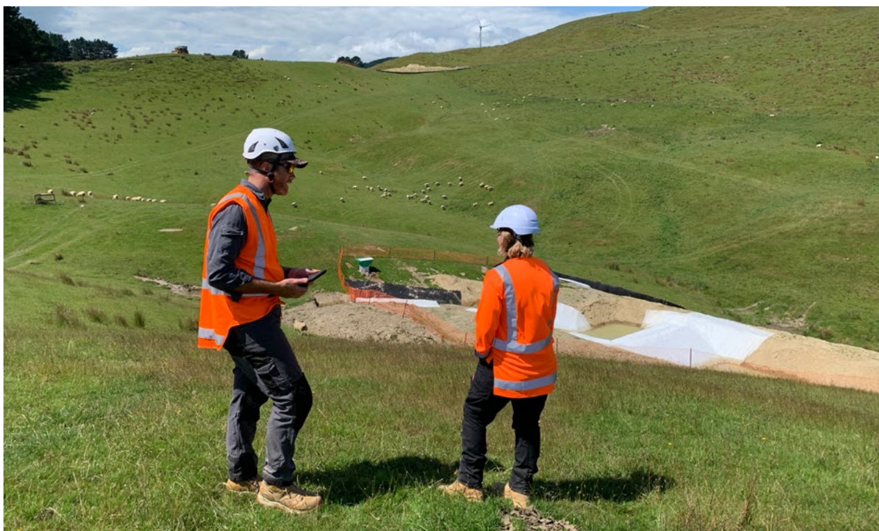
Regulatory staff inspecting a site
