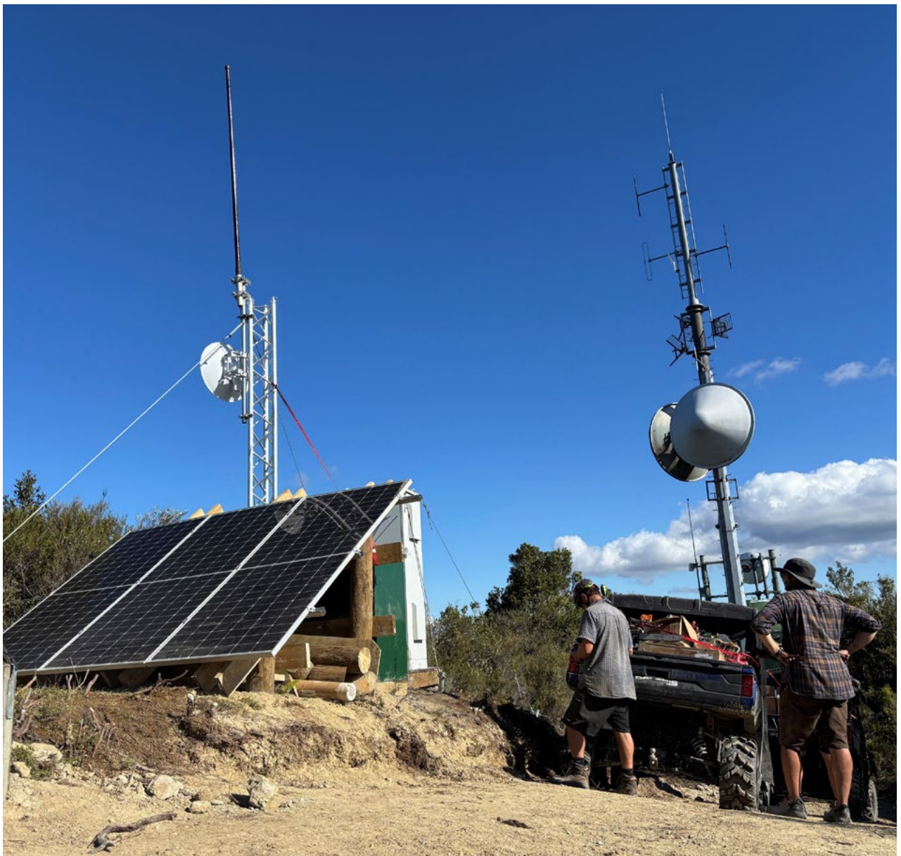
Installing environmental data monitoring equipment
