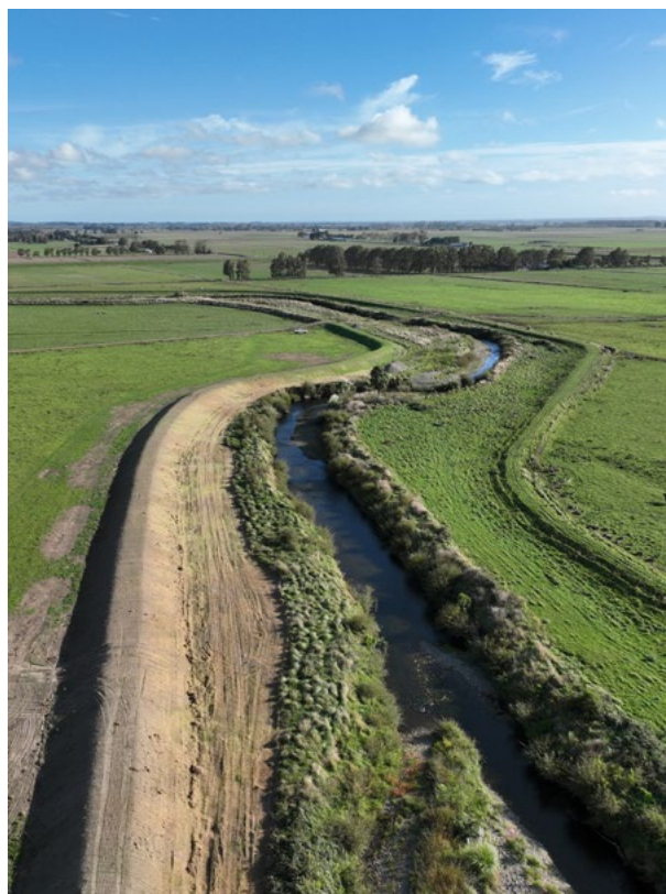
Newly built stopbank to provide flood protection
