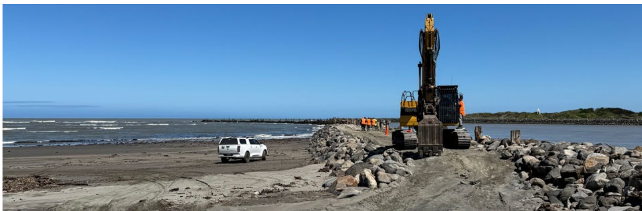
Digger at South Mole, South Mole
